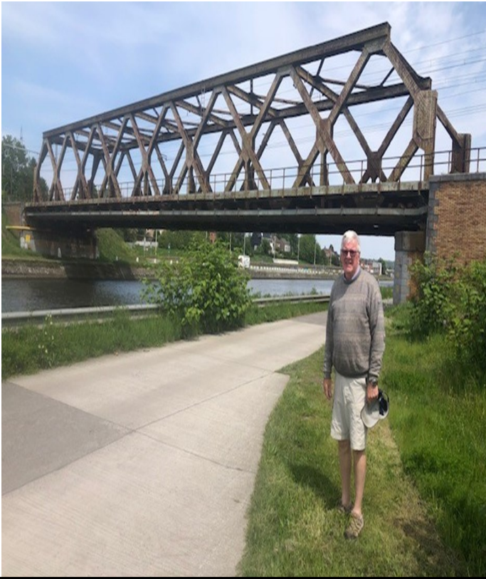
Nimy Railway Bridge, Mons.
